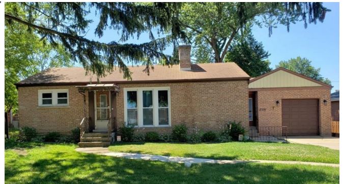
Edward Cabalan attached a breezeway and one-car garage to his ranch home on Lonquist Boulevard in late 1950. The home, which had been built the previous year, has since been torn down.
