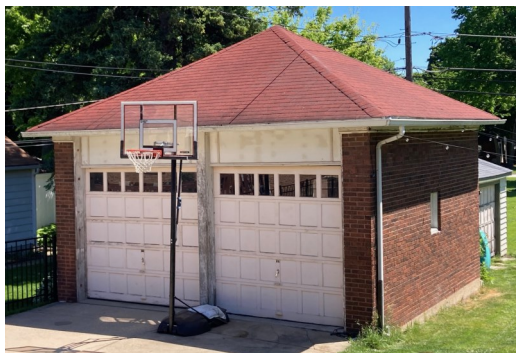
George and Selma Neitzke added this garage to the rear of their South Maple Street lot in 1929, six years after they built the home. They originally ran a produce market from it.
